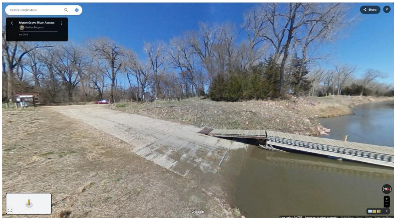
Current boat launch and view downstream from Myron Grove River Access.
